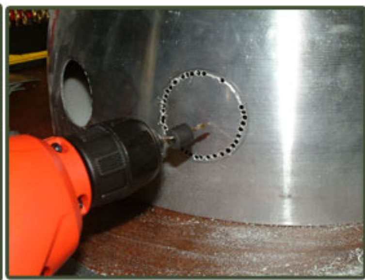
Drilling Holes in the Inner Dome
